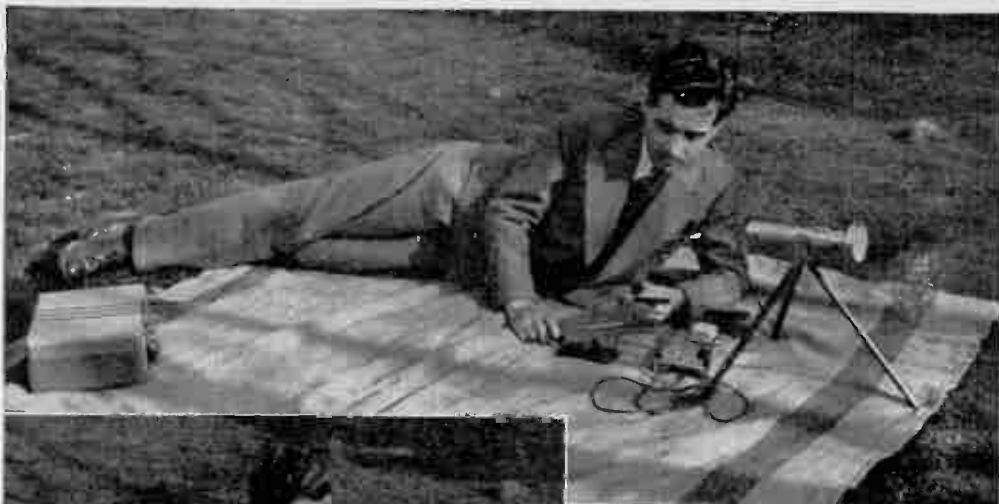
The operator taps out a code message on an ordinary telegraph key. Below he sights along the barrel to aim the flash light
