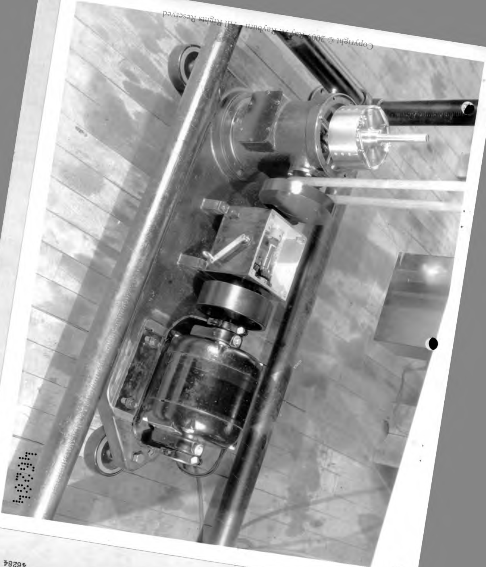
Sully Recording Machine - Motor and Drive Unit
