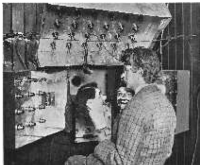
FIG. 91.—Bank of Lamps.
