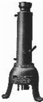
FIG. 38.—The Langmuir Mercury Vapour Pump.
