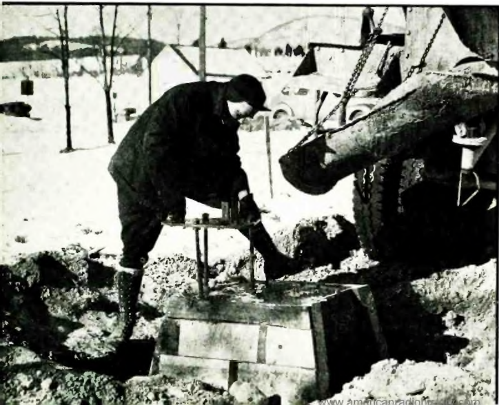
Fig. 8. The assembled base plate and anchor bolts, ready to put in place
