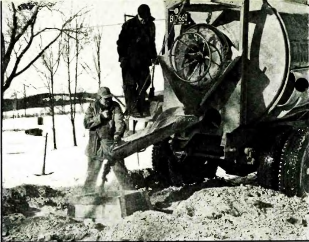
Fig. 7. Pouring concrete into the form for the base of the tower
