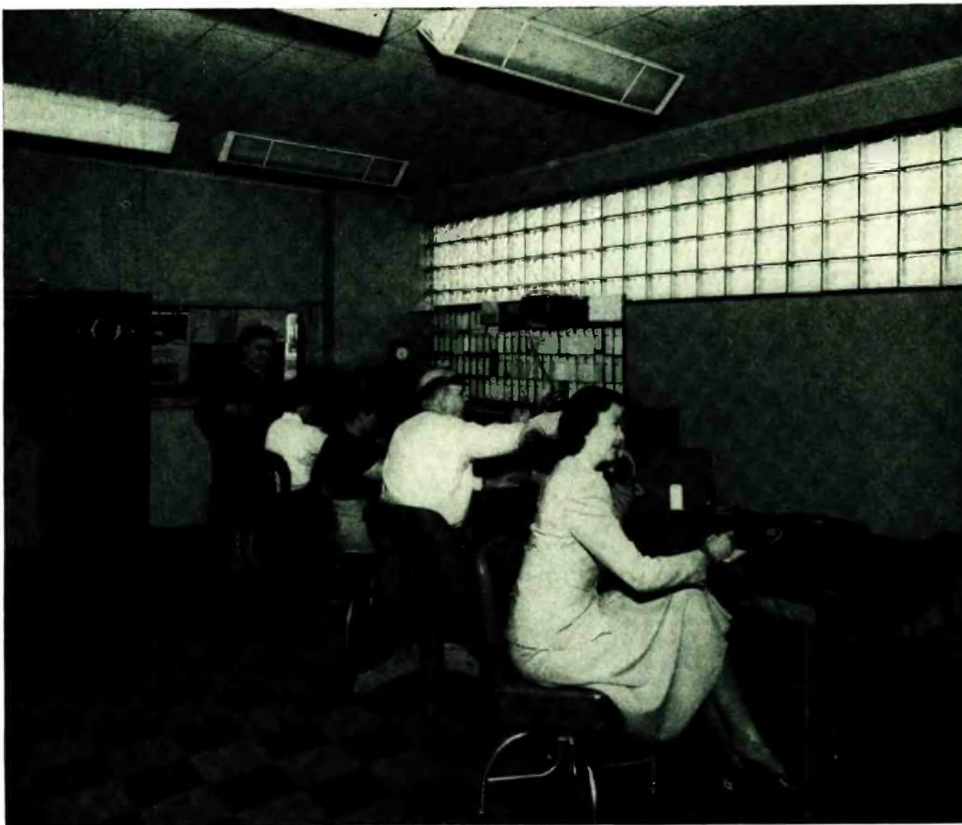
Fig. 3. A dispatching office for handling taxicab communications. This is a Motorola installation, operated by the Erie Cab Co.
