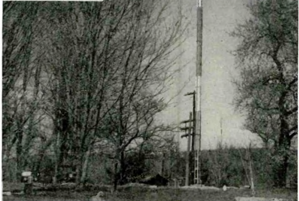
Fig. 17, above. The mount of the mast permits it to be lowered for attaching antenna rigs, or for changing the lights. This has proved to be a very satisfactory arrangement.
