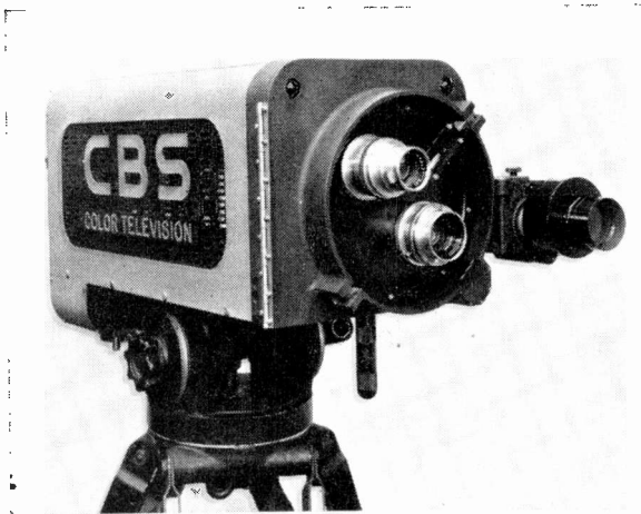
Fig. 4.—CBS color camera for use with CBS color television system.
