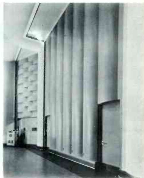
Figure 14-3 Vertical Poly-Cylinders. Note the control room window at the lower left of the picture.
