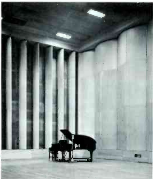
Figure 14-1 Vertical Tiltable Panels, and Poly-Cylinders on a Radio Studio Wall
