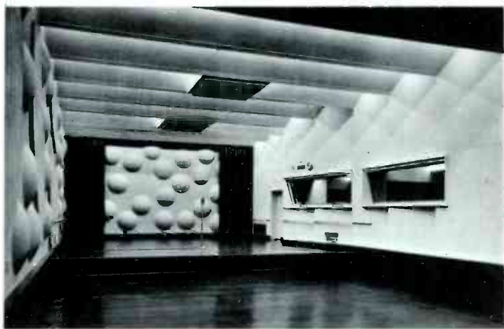
Figure 14-4 Audience Type Radio Studio. Observe how the walls and ceiling are treated to eliminate parallel surfaces. Note too, the control room window at the right, with a clock and loudspeaker above it, and the microphone receptacles located both below the window, and across the stage from it.
