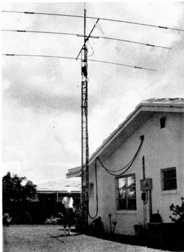
15-13. An ideal antenna for a small house and lot. The tower rises to 43 feet, telescopes to 20, and folds over. Antenna itself is a three-element, three-band beam for 10, 15, and 20 meters, with a short vertical rod at the top for 2 meters. Cables on side of house connect to beam and its rotator (dark area under antenna boom).
