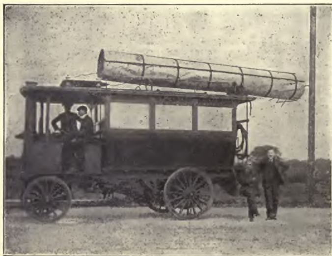
FIG. 259.—MARCONI CYLINDRICAL AERIAL.
