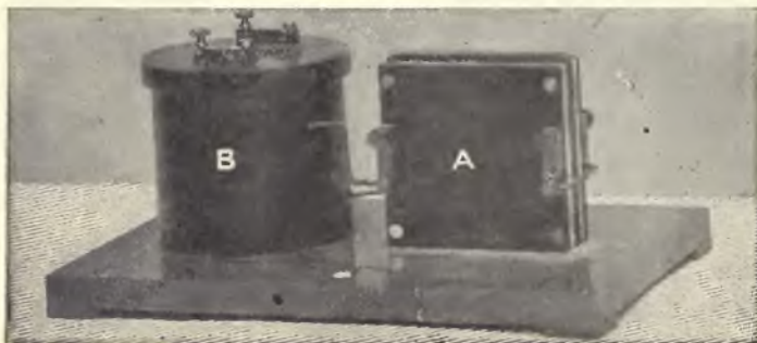
FIG. 231.—BRAUN CONDENSER AND TRANSFORMER.
