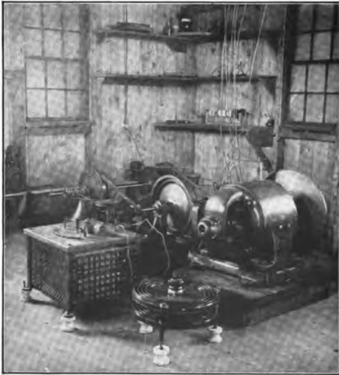
FIGURE 119 —Early form of Alexanderson alternator under test at Brant Rock Station of National Electric Signaling Company.
