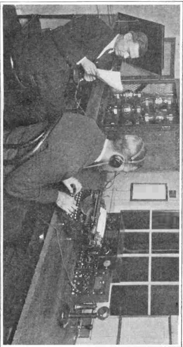
The "announcer" of a radio-phone broadcasting station, and the receiving operator. The announcer speaks into the microphone transmitter which he holds in his hand. Alongside of him is the radio-phone transmitting apparatus, with the vacuum tubes for generating and modulating the radio waves. This is WJZ, the Newark radiophone.
