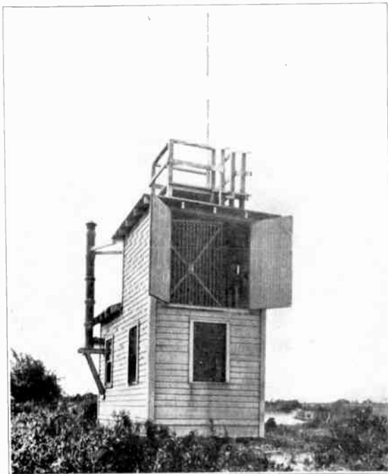
SANDY HOOK RADIO COMPASS STATION Showing the loop antenna above the operating room.
