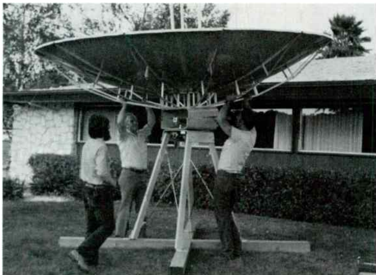
Fig. 11-12. Dish is lifted by backribs and placed on the mount.
