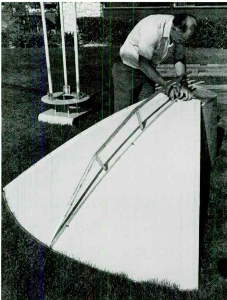
Fig. 11-6. Pedals of dish are affixed to backribs using garbage can for support. Note assembled center assembly in rear.
