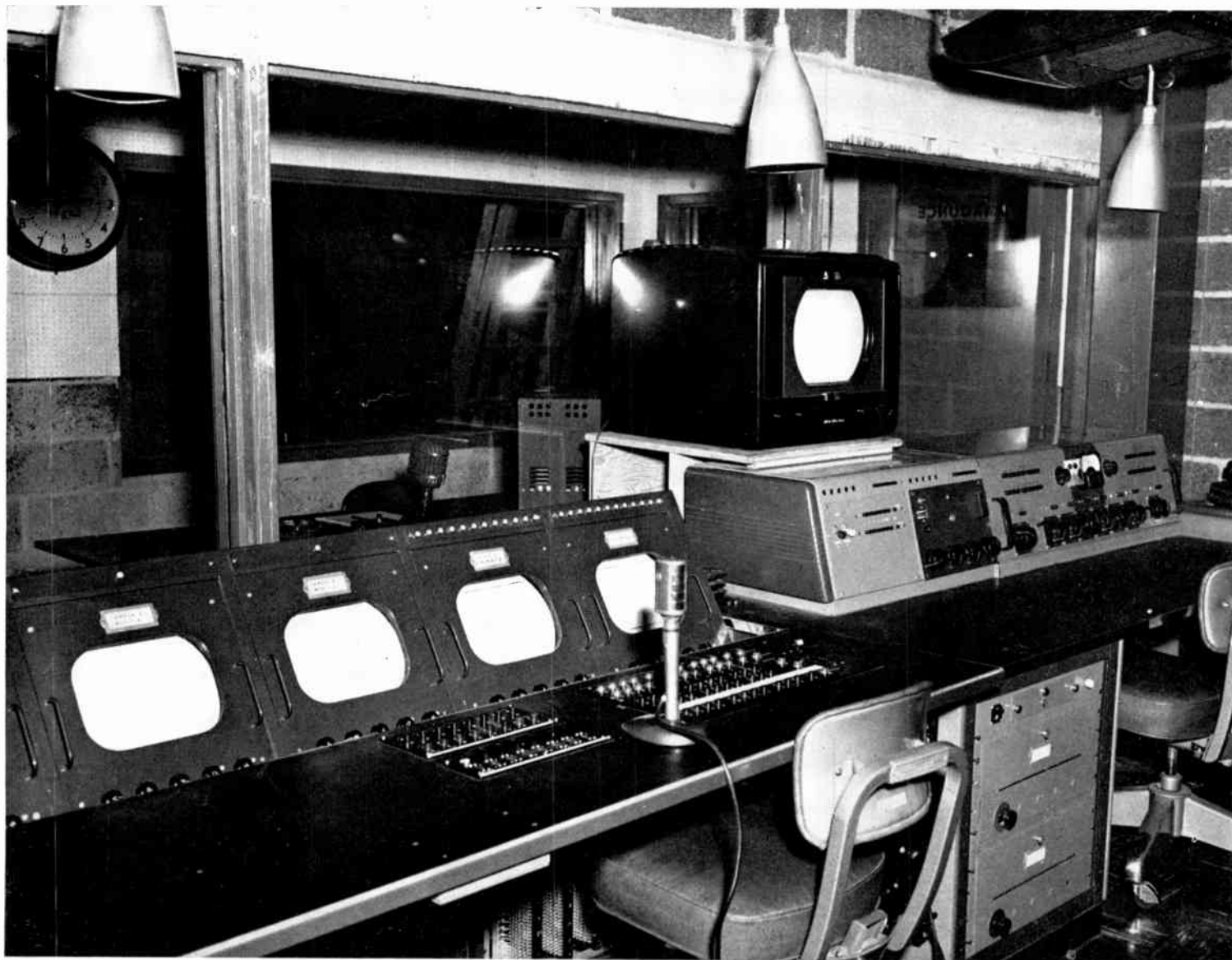
FIG. 15 (below). View of Control Room "C" showing arrangement of technical equipment. Program Director's Console with switching facilities is at left and Audio Console at right.
