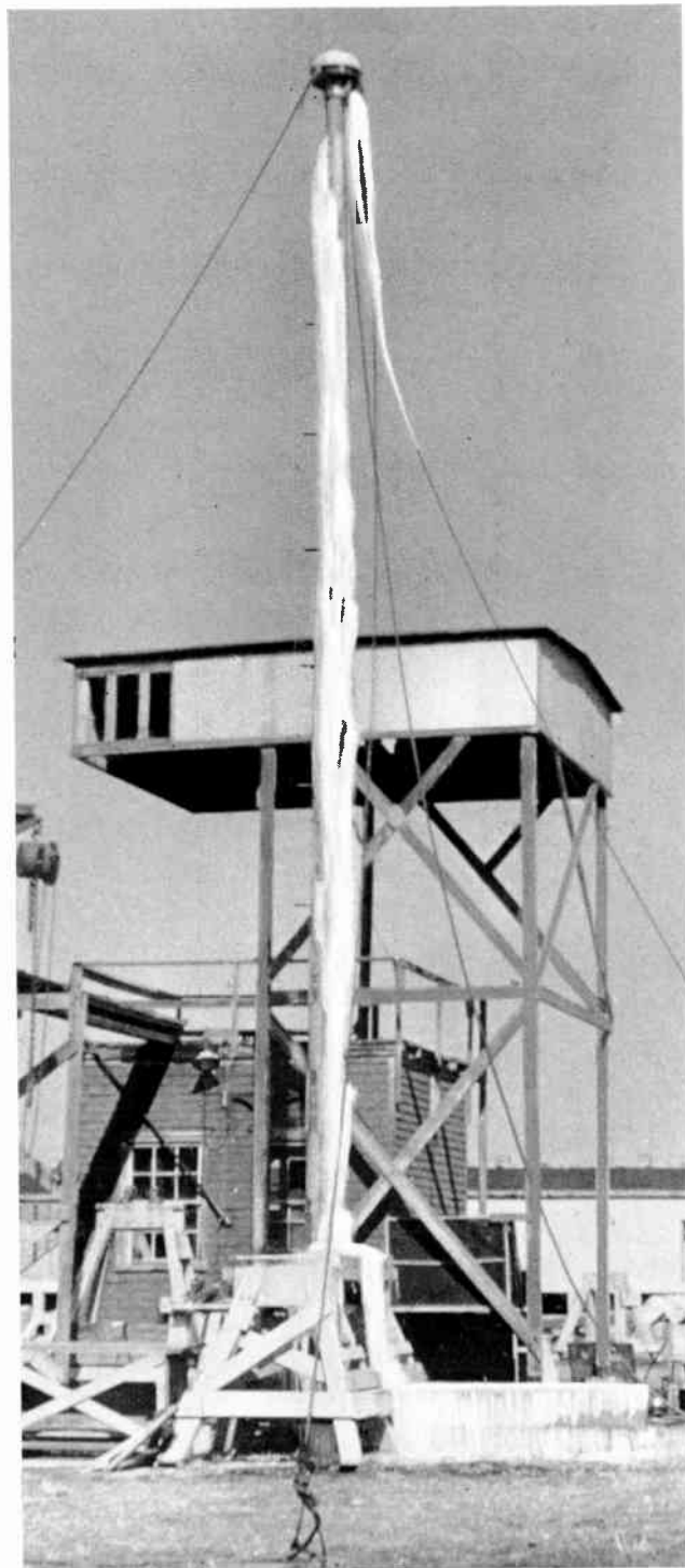
FIG. 13. Test set-up to study the effect of icing conditions on the RCA UHF Pylon Antennas.
