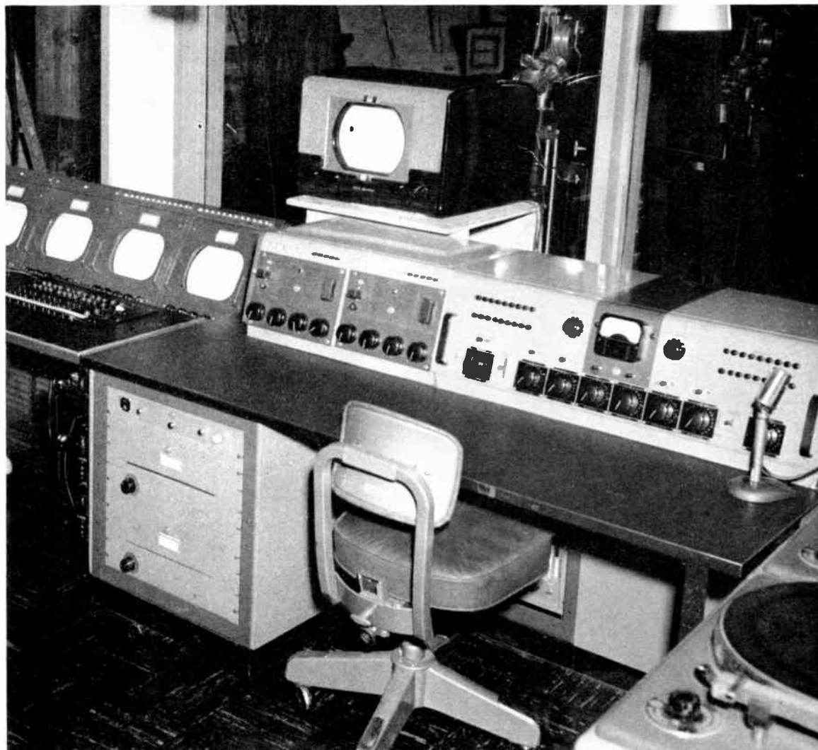
FIG. 20. Partial closeup view in studio "B" control room showing the audio control setup. Facilities consist of an RCA 76-B Console which is supplemented by two RCA OP-7 Mixer Amplifiers.
