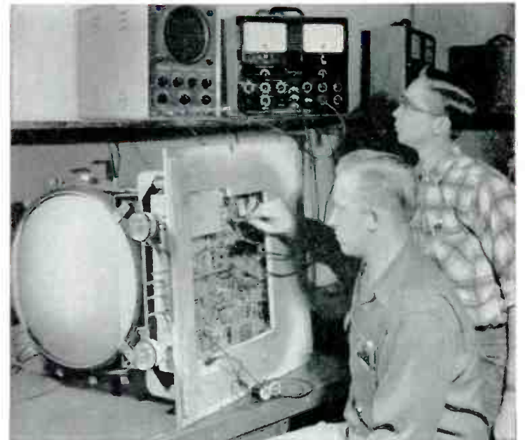
These students are performing a Color IF Alignment job on a Color TV Receiver using a sweep generator, marker generator and scope. One student is making adjustments while his partner is observing the scope pattern.
