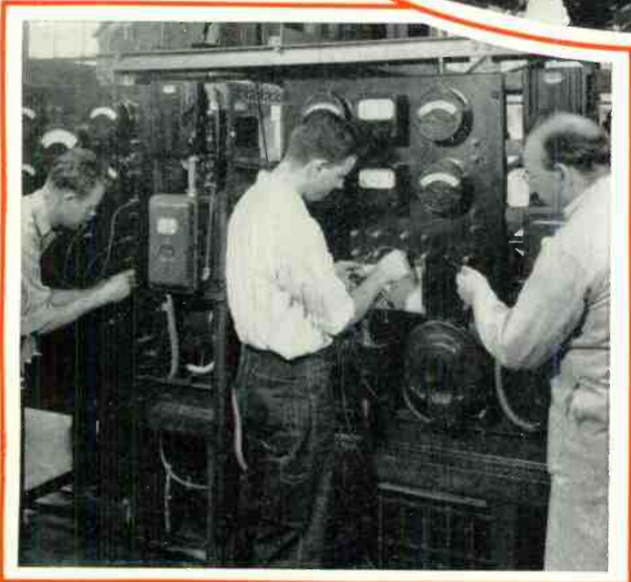
Here you see students making Power Factor and Efficiency test for three phase induction motor. These tests are used to determine horse power output of motor and Power Factor correction necessary to obtain minimum power rates.
