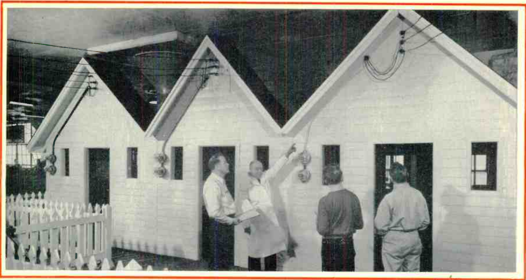
This is a picture of a Model Framework of a Bungalow which has been set up for students to get training under similar conditions as they will find out in the field. Here you see students getting instruction on the proper installation of a Service and Meter System.
