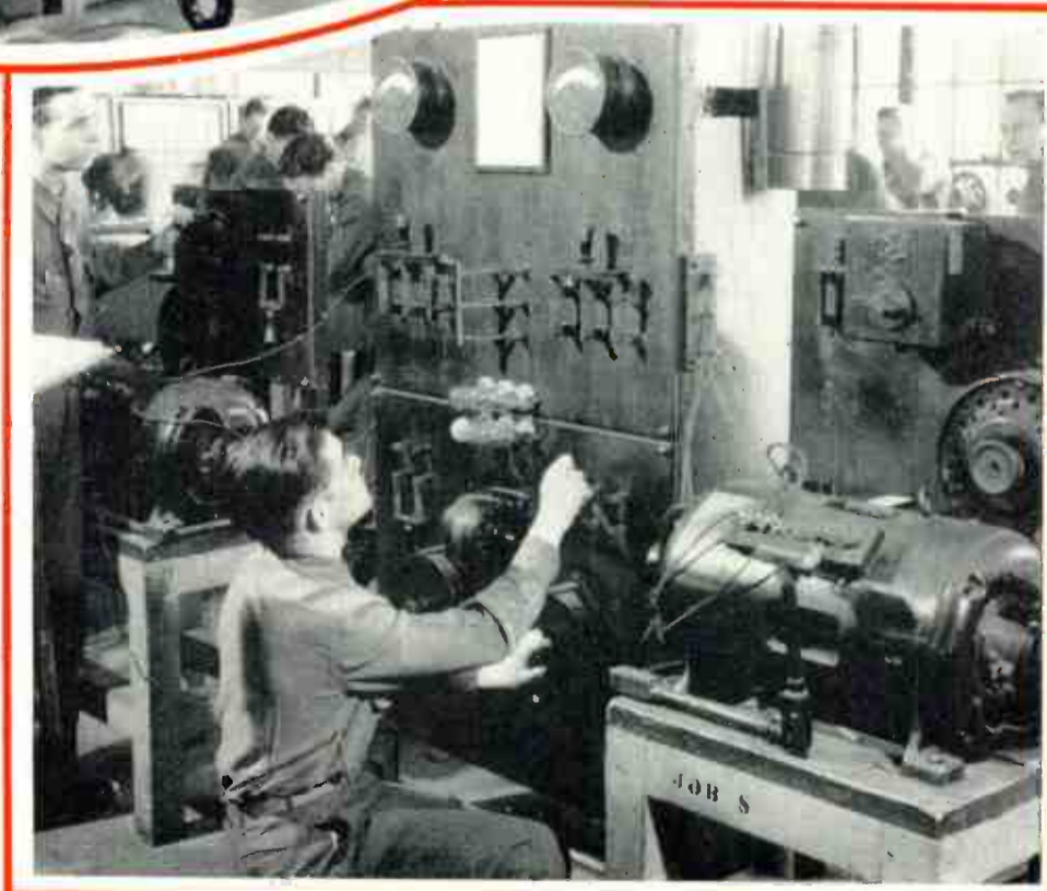
These students are getting practical instruction in the use of Lamps and Meters employed to synchronize A. C. Generators.
