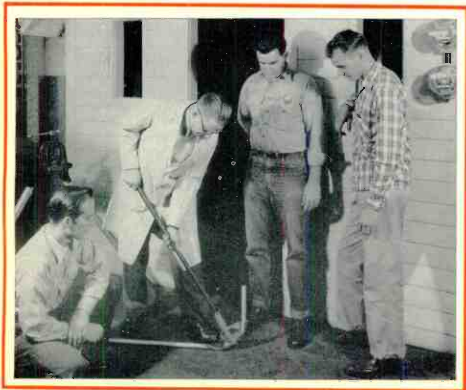
This instructor is giving a demonstration on handling EMT (Electrical Metallic Tubing). Much of the modern wiring for Light and Power is run through "thin wall" tubing of this kind. This training is designed to prepare graduates for work in the wiring of houses, buildings, etc.
