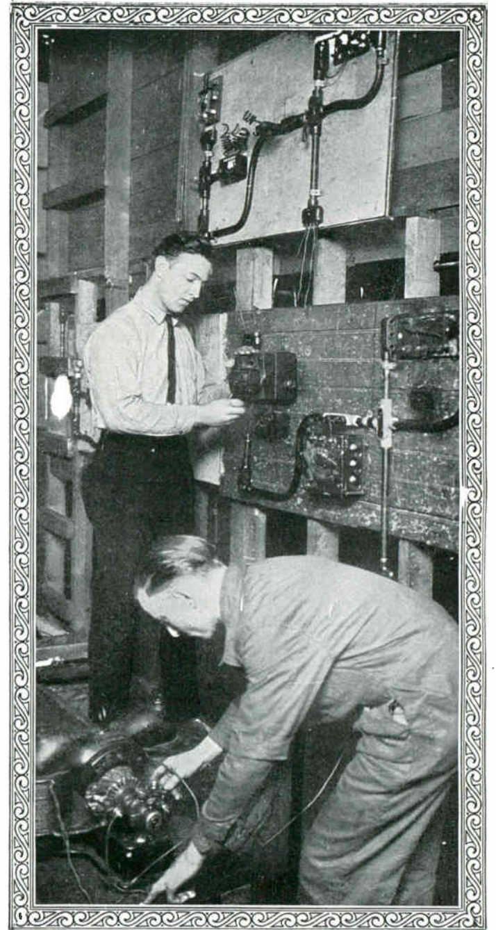
Motor Wiring and Installation
