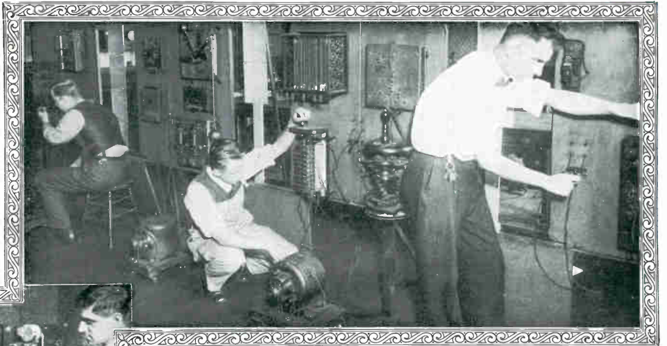
Operating All Kinds of Motor Control Apparatus
