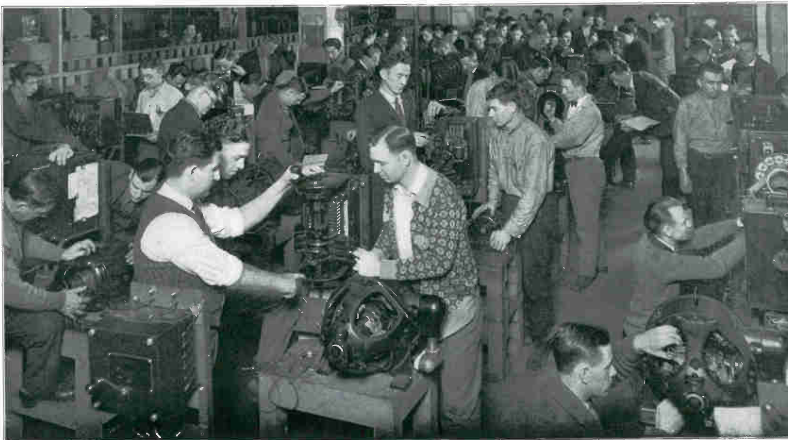
Students Wiring Up and Operating Various Types of D. C. Control Apparatus and Motors
