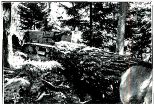
Fig. 25. This photo shows a Diesel-tractor used for dragging out logs in the lumber woods. (Courtesy of the International Harvester Company.)
