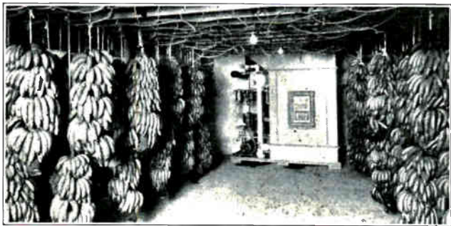
Fig. 5. Interior view of a refrigerated room used for cooling and storing fruits. Note the refrigeration unit in the background. Courtesy York Ice Machine Corporation.
