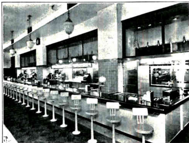
Fig. 8. Interior view of a modern air-conditioned lunch-room. Note the air delivery ducts and openings along the ceiling. Air-conditioned eating places are much more popular and generally do a much greater business than those that are not so equipped. Courtesy York Ice Machine Corporation.
