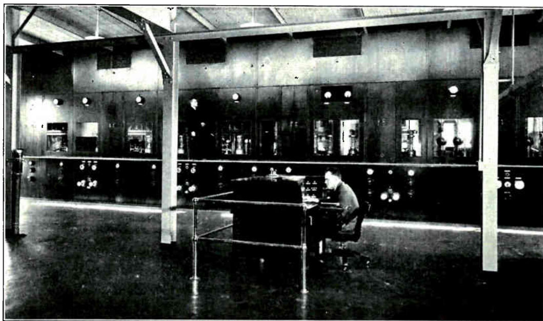
Fig. 1. Main transmitter panel of WLW, Crosley Radio Co.'s large 500,000 watt broadcast transmitter. Only men with thorough training and a good knowledge of electricity and Radio are qualified to operate a station such as this.
