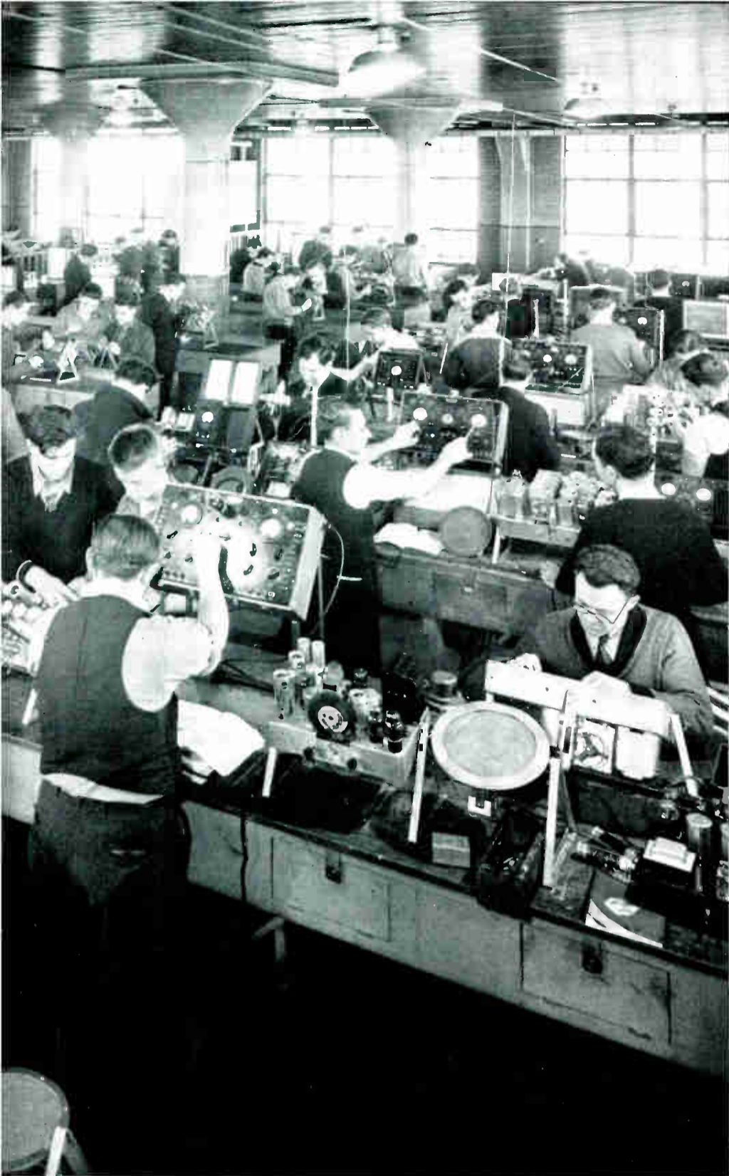
Above is an interesting view of part of the Servicing Dept. showing students using modern analyzers to locate troubles in various types of A.C. receivers.
