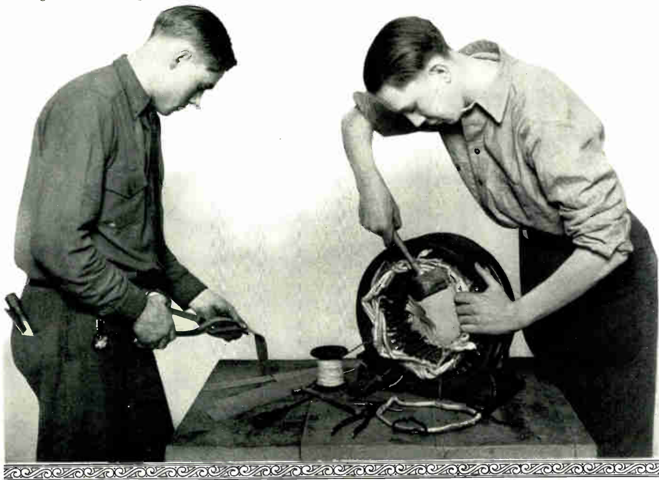
Overhauling and Testing a Motor Before Rewinding
