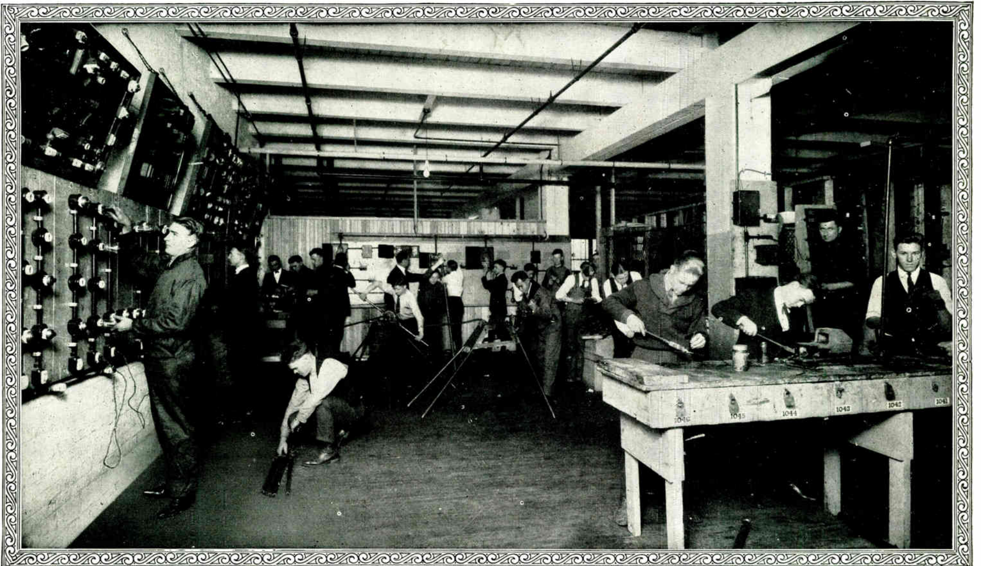
Another Partial View of the Construction Department Showing Bending and Threading Conduits, Soldering Connections and Switching Work on Concealed Circuits Boards
