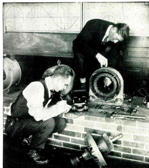
Students Testing Induction Motor
