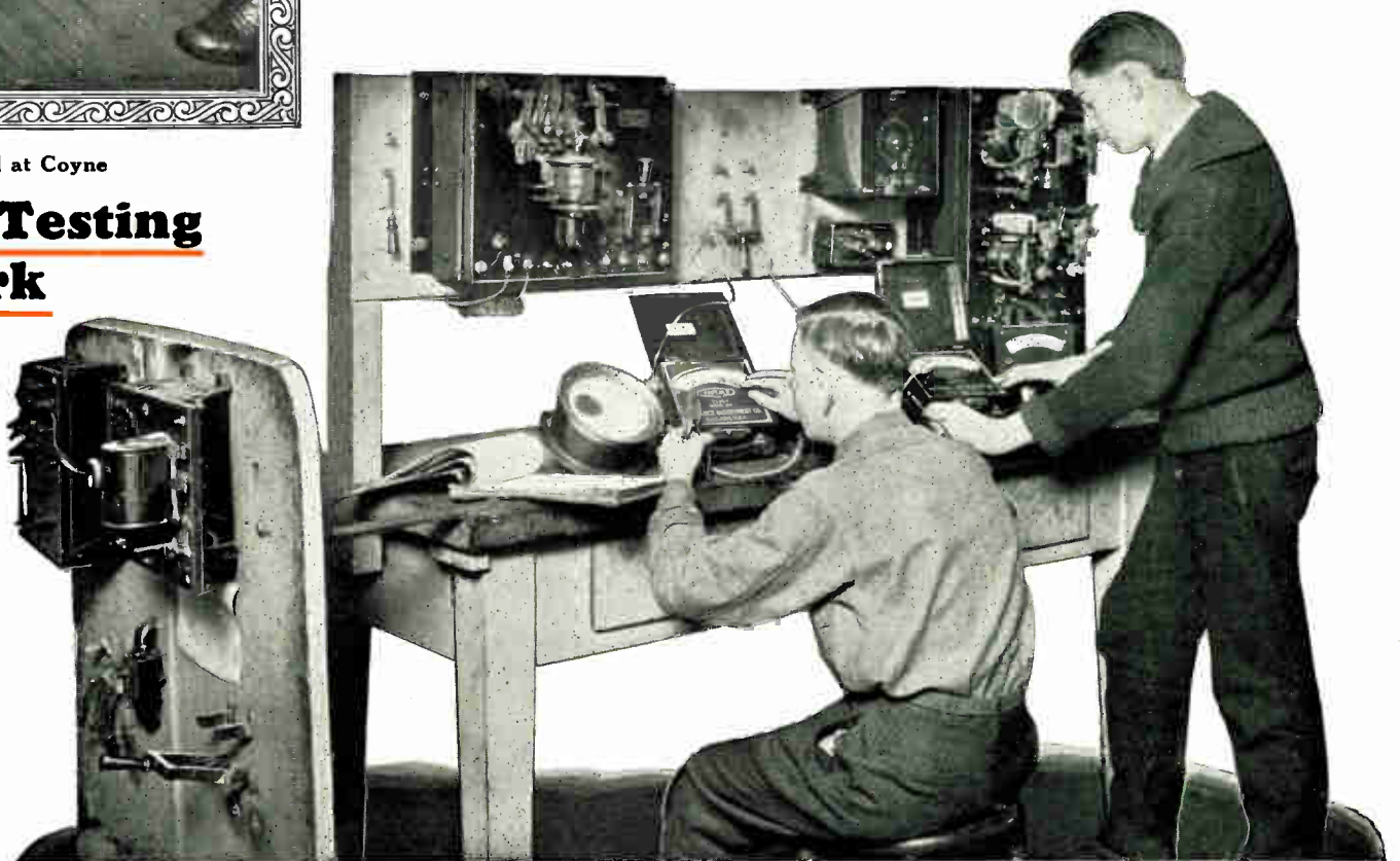
Students Testing Automatic Elevator Control Apparatus
