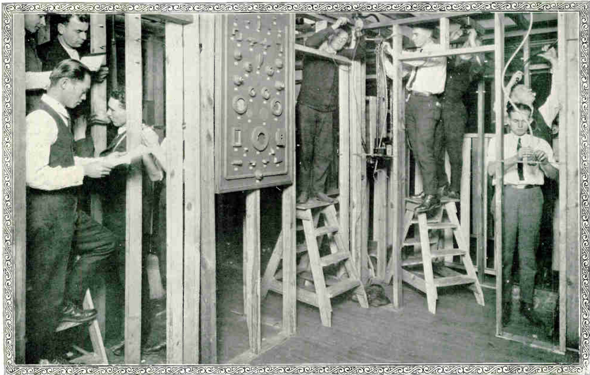
House Wiring—Showing B. X. Work—Just Like You Do It Out on the Job
