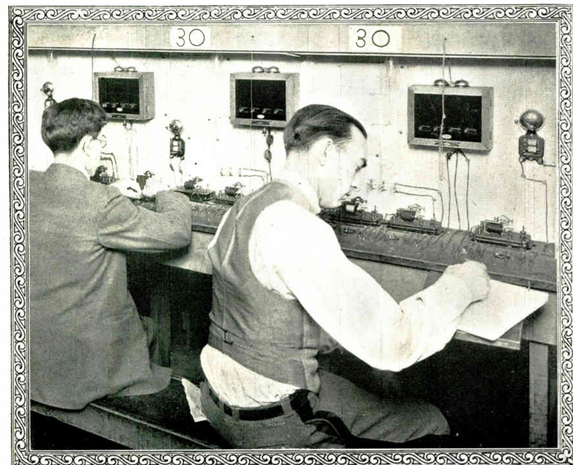
Wiring Burglar Alarms in Circuit Department. Note That This Is Job Number 30
