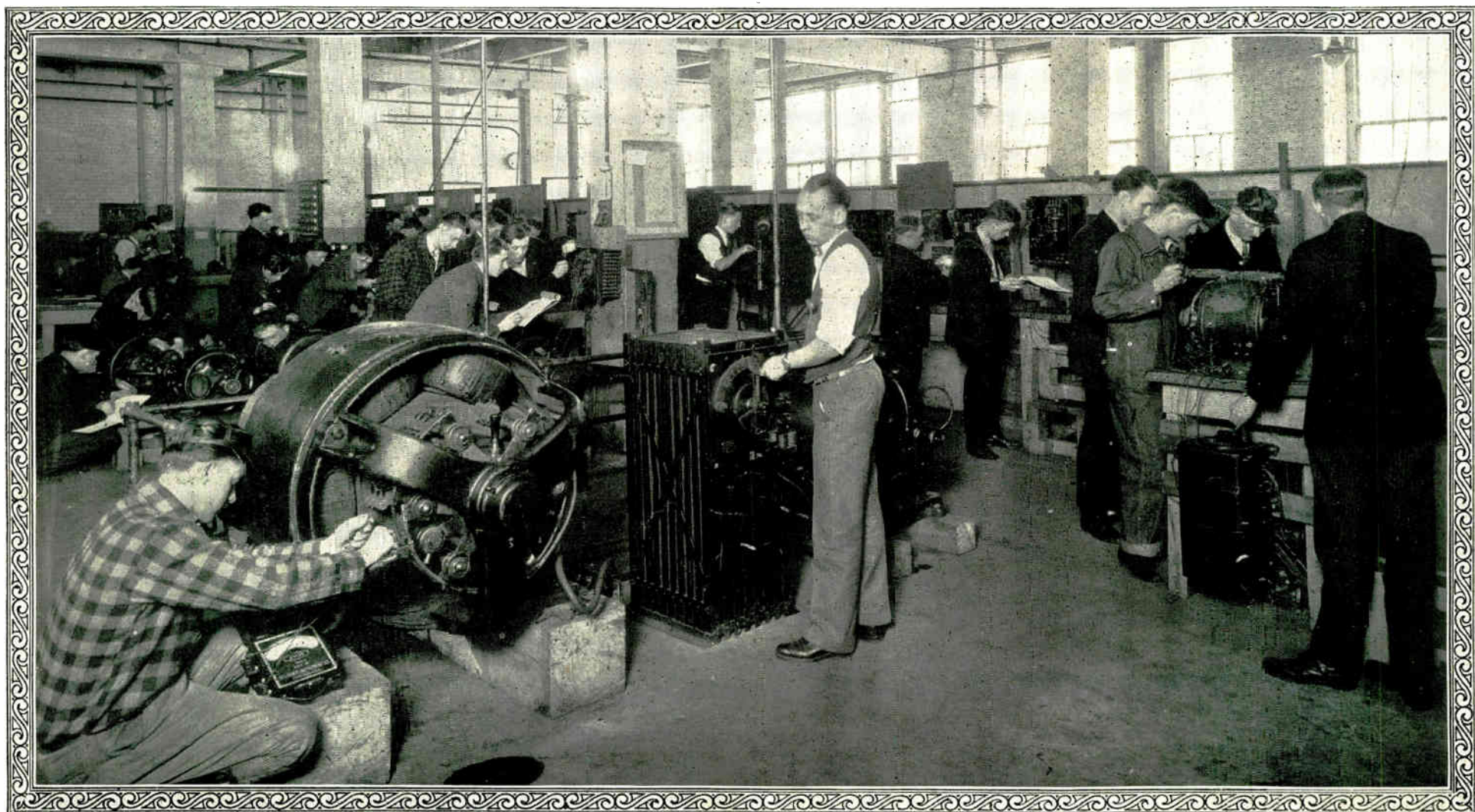
A General View of a Small Section of the Direct Current Department Showing Part of the D. C. Apparatus
