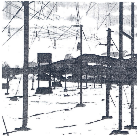
The Swiss Antenna System.
