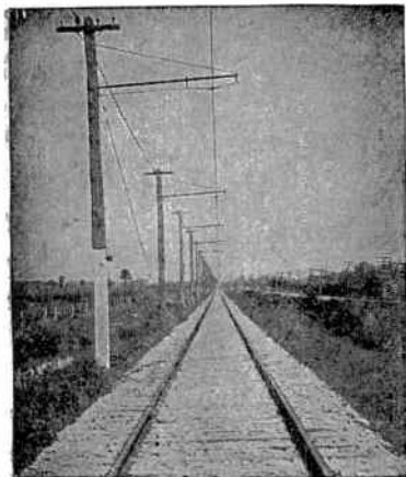
Figs. 3,499 and 3,500.—Overhead construction on the Indianapolis & Louisville 1,200 volt line. The line throughout is of the single bracket construction on tangents, as shown in fig. 3,499 and of the span type at curves, as in fig. 3,500. The poles are spaced 90 ft. apart on tangents and 60 ft. on curves. A single No. 0000 trolley wire of grooved section is used, and is held in alignment by 8 in. four screw clamps reinforced with soldered strain guys every half mile. Lightning arresters are installed every 1,000 ft., and are tapped alternately to the trolley and feeder. Telephones have been installed throughout the system, and jack boxes are attached to the poles at all sidings and at half-mile intervals.
