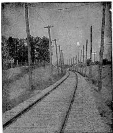
Figs. 3,499 and 3,500.—Overhead construction on the Indianapolis & Louisville 1,200 volt line. The line throughout is of the single bracket construction on tangents, as shown in fig. 3,499 and of the span type at curves, as in fig. 3,500. The poles are spaced 90 ft. apart on tangents and 60 ft. on curves. A single No. 0000 trolley wire of grooved section is used, and is held in alignment by 8 in. four screw clamps reinforced with soldered strain guys every half mile. Lightning arresters are installed every 1,000 ft., and are tapped alternately to the trolley and feeder. Telephones have been installed throughout the system, and jack boxes are attached to the poles at all sidings and at half-mile intervals.
