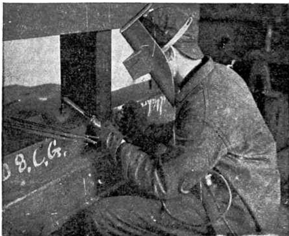
Fig. 4,501.—Operator using C and C electric arc welding metallic electrode. The electrode itself is melted and supplies the extra metal necessary for welding or building up.
