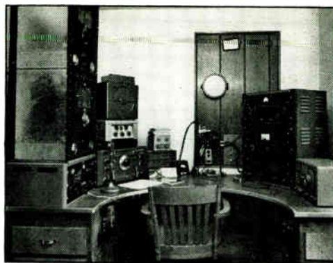
One of the most convenient station arrangements is to build a semicircular operating table as shown here. All operating controls are readily available, and considerably more equipment can be grouped around the operator than when an ordinary desk is used. ( W2SAI, Riverton, N. J. )
