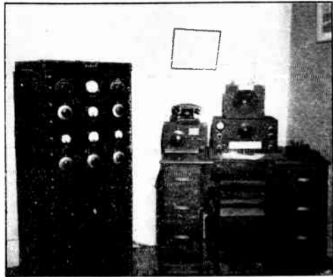
This 700-watt station is tucked away in one corner of an apartment. The secret to a compact station is to do away with frills not necessary for communication. The transmitter and supply are in the cabinet, the VFO and receiver on the table. (W2AIO, Rutherford, N. J.)
