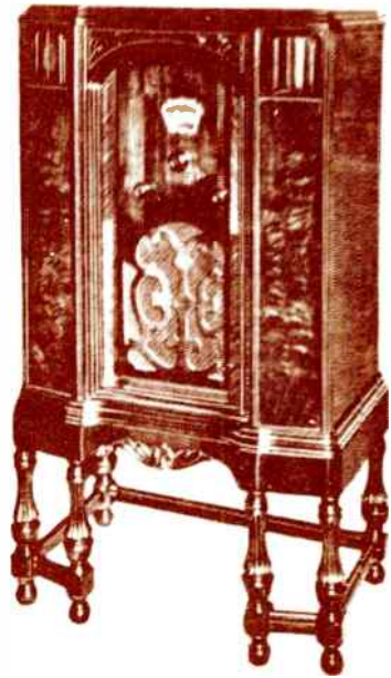
Grebe 84. Six legged console with sliding doors of matched Oriental walnut. Pilasters of two piece highly figured Butt walnut. Chassis is the 8-tube Superheterodyne used in Model 80. Equipped with 17" dynamic speaker. List Price $89.50 complete. Tax Paid.
