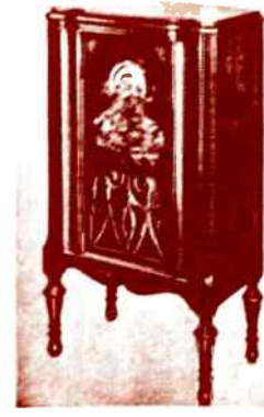
CLARION 81, $84.50 Superhet., 7 tubes with var-mu and pent.
