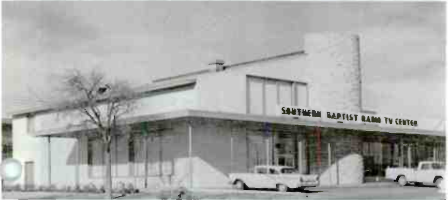
6248 Camp Bowie Blvd., Fort Worth, Texas—second home of Radio-TV Commission
