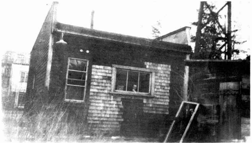
Rear view of the CBC Prince Rupert establishment.
