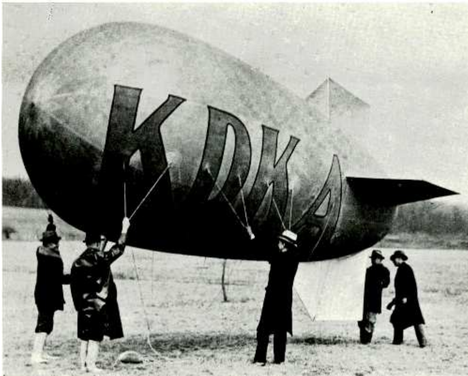
An experimental antenna carried aloft by a balloon was tried by KDKA at Saxonburg, Pennsylvania. The balloon later pulled away from the antenna, floated up and was destroyed.
