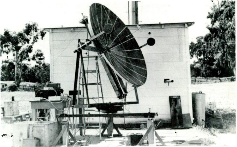
The first microwave radar apparatus using klystrons. Prior to 1941, this was tested on the Stanford campus by aiming at a rented airplane. Klystrons are directly behind the "dish."
