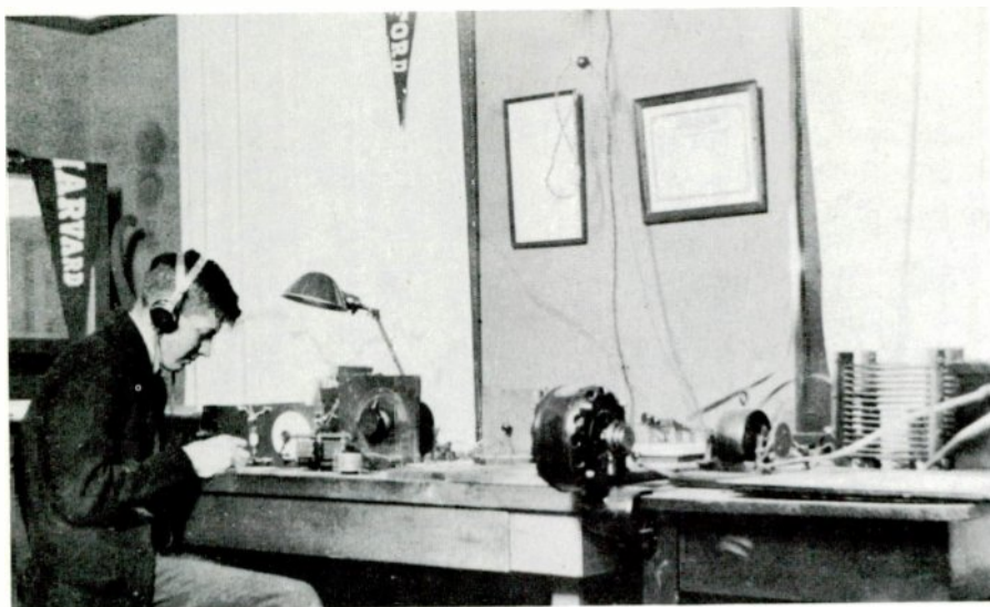
Three of the Bay Area "hams" who became nationally known in electronics. Above, Frederick E. Terman in 1917 with spark gap transmitter, crystal detector, one-tube amplifier. He listened to voice from Herrold's San Jose station and to code from others as far away as Fred Roebuck in Phoenix, Arizona, before Fred moved to California.
