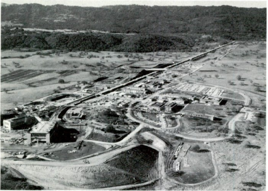
Aerial view of the Stanford Linear Accelerator on university land west of the main campus. Electrons begin their journey at end at right background, race two miles to smash the targets in buildings in left foreground. Note the many other buildings necessary for the project.
