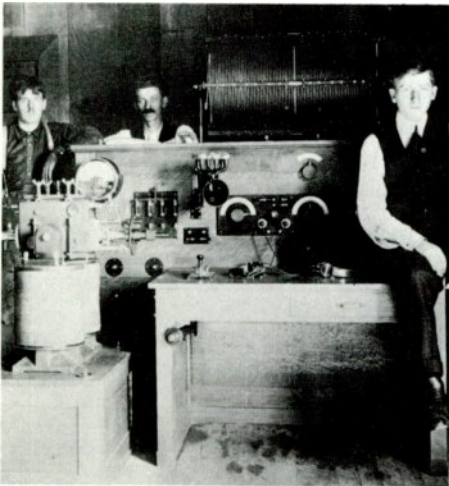
(L to R) Douglas Perham, C. Albertus, Peter Jensen with 5 kw Federal-Poulsen arc station equipment, about 1910. Arc is mounted on box at left. Note tuning knobs and multiple-unit microphone above telegraph key on operator’s table. Drawing is a later 30 kw arc, about 4 ½ feet tall. Jensen became co-inventor of the loudspeaker. (See Ch. VI.)
