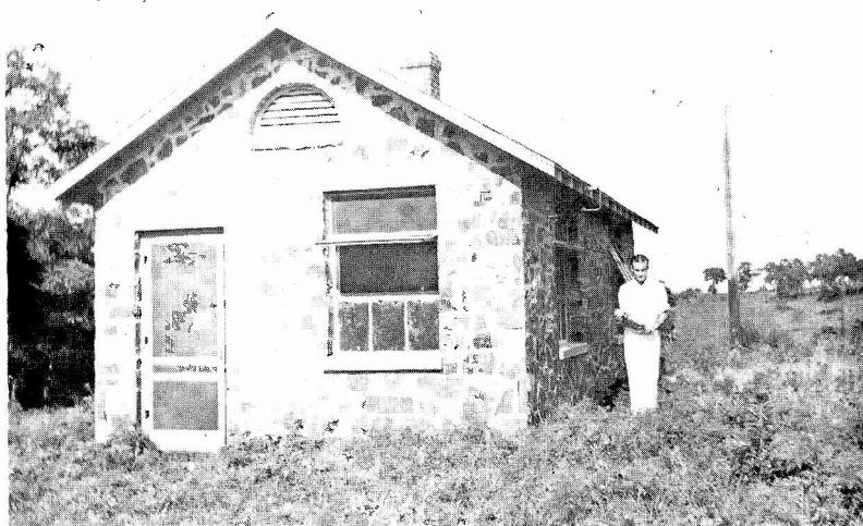
The KUOA transmitter building on Mt. Sequoyah in 1934. Engineer Lester Harlow holds a Type 851 transmitter tube used in the final amplification.
