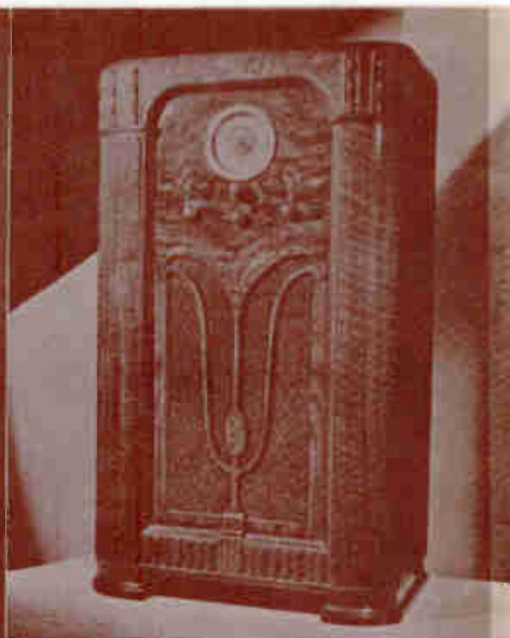
7-tube Ferradyne Round-the-World receiver with all metal tubes. New Diffusalite Magic Dial.
