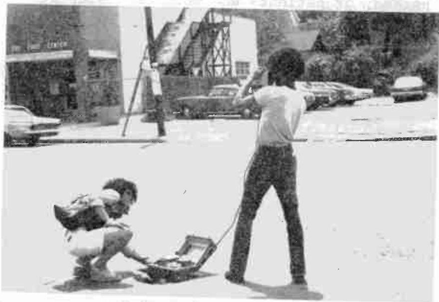
3-30 The outside of the building is also taped.
