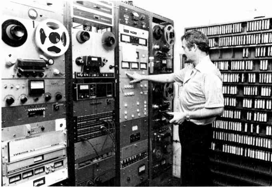
11.10. Among other duties, the engineer is responsible for checking the transmitter regularly and noting the readings on a special form for the FCC. It is vital that stations do not exceed their power and frequency allotments. Several have lost their licenses for such violations. Photo by Nadine Ohara. Courtesy, KSFO radio, San Francisco.
