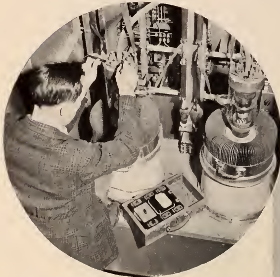
Transmitter tube measurements being made by an RCA engineer in high-power broadcasting station.
