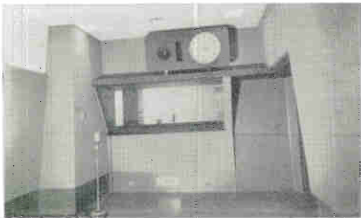
Looking forward into the control booth of a small studio. Notice the mike in the booth and the speaker on the board with the clock. This mike and speaker are the director's talk-back through which he directs the program.
