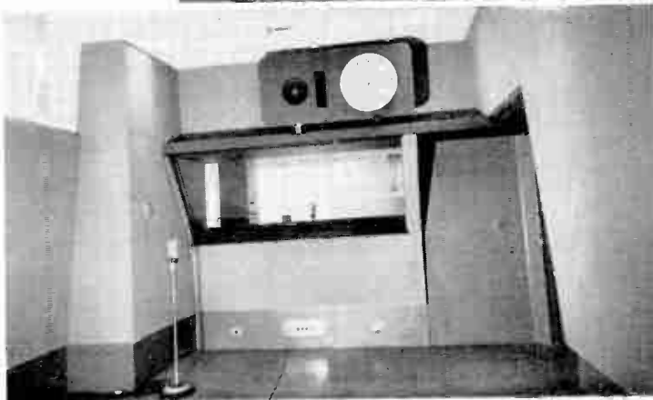
Looking forward into the control booth of a small studio. Notice the mike and the speaker on the board with the clock. This mike and speaker are the director's talk-back through which he directs the program.
