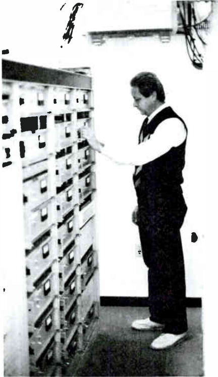
Figure 12.22 Cable system headend. A technician adjusts a control at Cox Cable-University City's headend. At left is the front of one rack of equipment; at right, the back of another—two of many that fill the small cement-block building. All signals feed to the box at top, the first amplifier in the system. From the other side of the amplifier emerges the trunk line, which carries programming throughout the franchise area.
