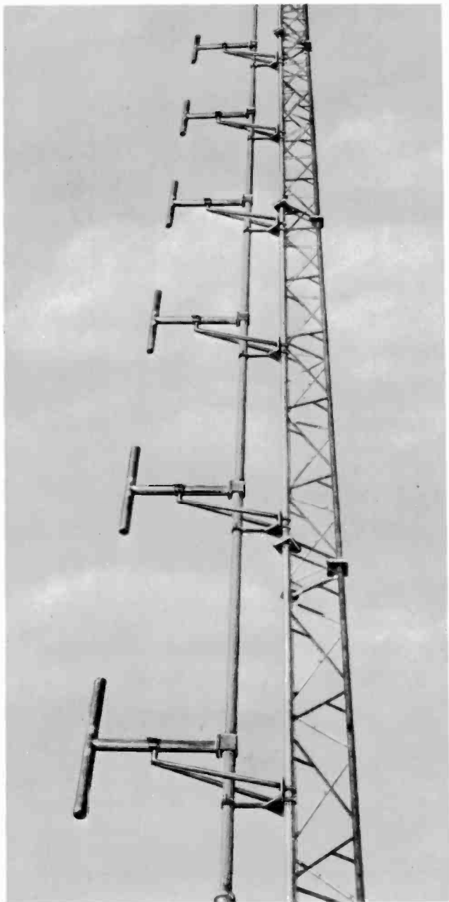
Fig. 8-4. Radiating element of a typical vertically-polarized FM antenna.
