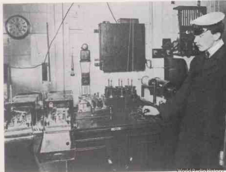
18 1900 saw the birth of The Marconi International Marine Communication Company Limited, whose purpose was to work an exclusive licence for all maritime purposes. More and more ships were being equipped, and the photograph shows a typical installation of the period. At this time, also, Marconi took out his famous Four Sevens Patent for tuned coupled circuits.
