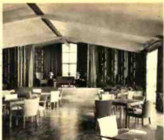
IN THE CENTRAL BUILDINGS are located the dining room, lounge, library, administrative offices, kitchen and laundry, all blazingly modern.
