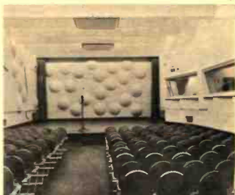
NEW YORK, N. Y. — NBC — Very ultra is 6D, NBC's newest Radio City broadcast studio. It embodies many novel and distinctive features in design—such as sawtooth shape of ceiling and bubbled stage wall.
