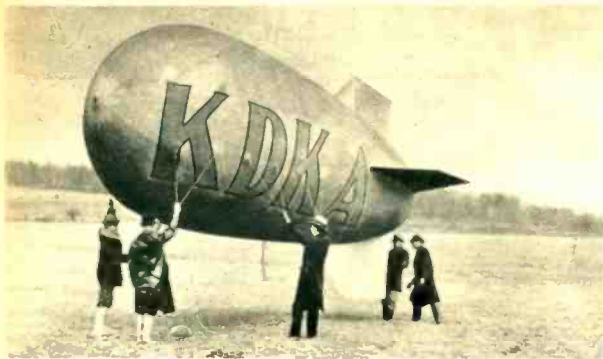
TODAY'S RADIO TOWERS were unknown, when Station KDKA tried to get height for its antenna by hoisting this balloon at Saxonburg, Pa. It eventually broke loose, and nearby farmers—spurred on by promise of a $25 reward for bringing it down—literally shot it to pieces!
