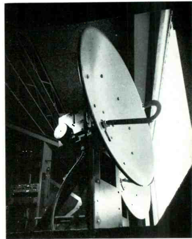
SIGNAL LINK • Most new stations microwave their signal to the transmitter site. Some (like WHEN-TV Syracuse) pamper their gear by housing it inside (above).
