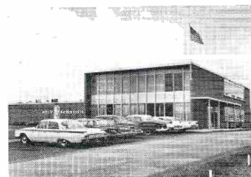
New Building for fast-growing Poly-Scientific Corp. at Blacksburg, Va. Many new industrial plants boost prosperity of WDBJ-TV coverage area.
