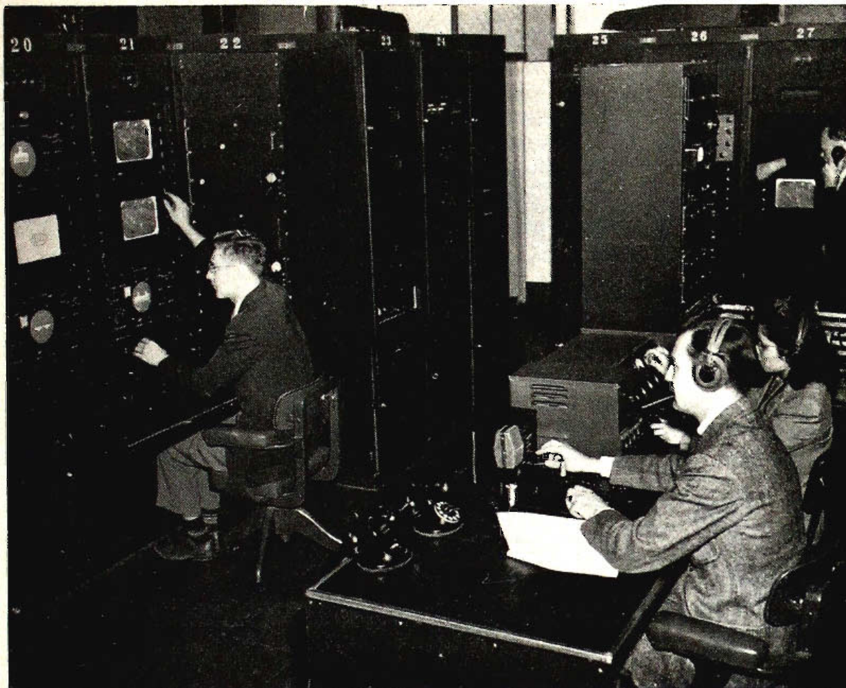
Master control of WPTZ is seen in action during football telecast. At video controls, left , is Farrell Quigley, a key staffer. In foreground is producer Paul Knight. Beside him is sound operator; in background, relay-receiver engineer.
