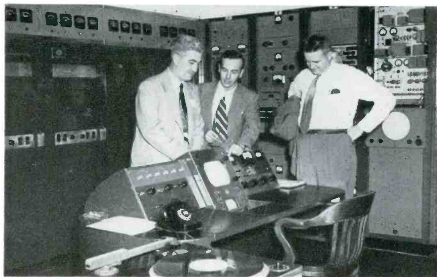
Figure 3 In the transmitter room at Bridgeport during uhf seminar visit, Dr. Roy Marshall listening to a report on the operation of the console which permits viewing of picture on 530 or 850 mc output or direct. Monitor at right also provides view of picture direct from WNBT in New York.
