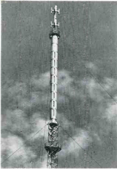
Figure 2 (Left) View of top section of 750' mast, showing the transmitting antenna, one side of a 4-sided vhf slot antenna which is for future use and, below the platform on the triangular section, a two stack receiving antenna.
