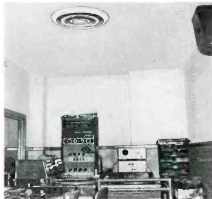
Below Control room at WPTZ with a circular air unit.
