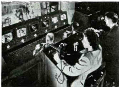
G-E control and monitoring consoles.
