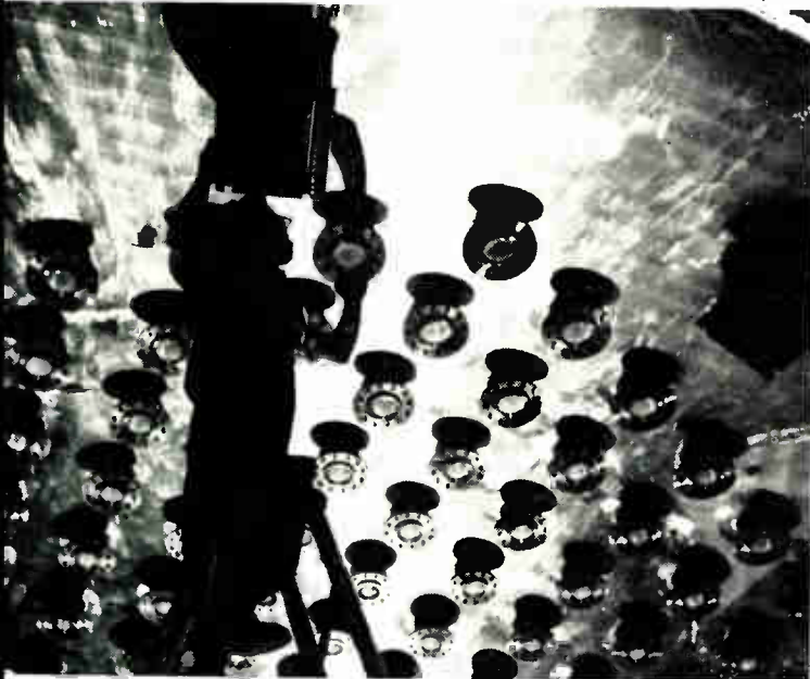
Giant pumps leading from one of two space chambers will be used to help evacuate the chamber as it simulates conditions of outer space. About half of the 58-foot-high chamber is shown here, the other half extends through to the floor below.
