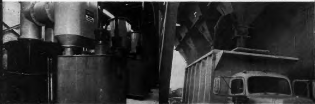
COMPACT HIGH VOLTAGE INSTALLATION. Westinghouse Silicon Rectifier Stacks are housed in Buell Transformer Rectification Unit (left rear). Tank (center foreground) is the separate Immersed Distribution High Voltage Switch Unit. An alternate Buell model encloses both units in a single tank.
