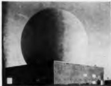
(Above) Automatic checkout and monitoring equipment for BMEWS uses punched cards and targets simulated on tape. (Below) Tracking radar is inside this 140 ft. dia. radome.
