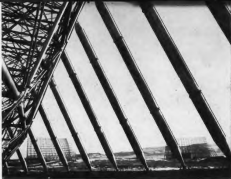
(Above) All installations at the radar site are connected by "covered highways." (Right) Surveillance reflectors were produced by D. S. Kennedy Co., designed by GE. 1,500 ton reflectors are supported by these 42 in. dia. backstays and trusses.
