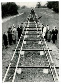
IT&T Corp. is sending live TV over half a mile through this 3 in. pipe at Hertsfordshire County, England. They are believed to be the first transmitted by circular waveguide or by pulse code modulation for such a distance. Even greater distances are possible with repeaters. In commercial use, the pipe would be buried.
