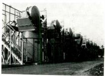
Nine SPC-55 radars, used with the Navy's ship-to-air TERRIER missile, are being tested at this facility operated by Sperry Gyroscope Co. at MacArthur Field, L. I. Testing program involves an area of over 100,000 square feet.
