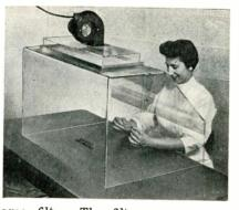
area filter. The filter removes airborne dust particles down to 0.5 micron in dia. and provides an internal "positive" pressure which pre-vents unfiltered room air from entering the open front. Working area measures 34 x 24 x 19¼ in. It is constructed of optically-clear, ¼ in. "Plexiglas." Air-Shields Inc., Industrial Division, Hatboro, Penna.
