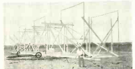
Directional antenna used by Karl G. Jansky in discovery of stellar radio signals at Bell Telephone Laboratories in 1932.
