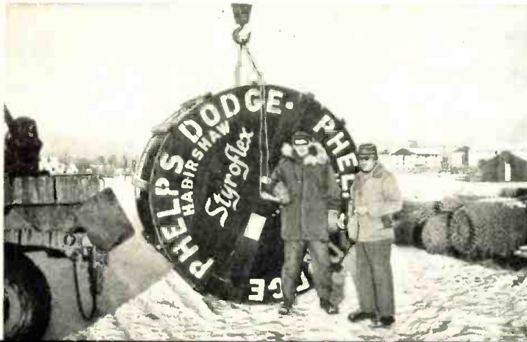
Styroflex reel is loaded on truck for transportation to installation site.
